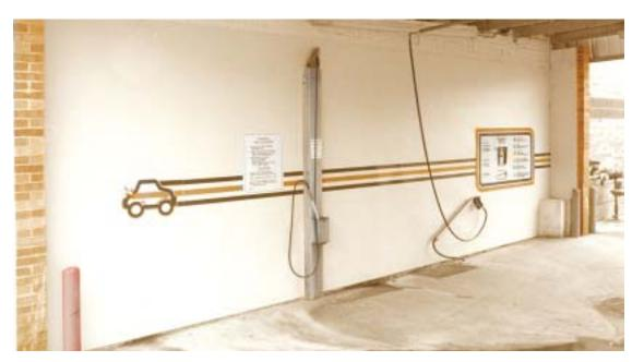
He used rivets only (no adhesive) to mount his panels. Ross said, "they're a little loose and flexible in places, but I like that because we get so much ice in cold weather. All I have to do it hit the panels and since they're a bit flexible the ice cracks and falls right off."
