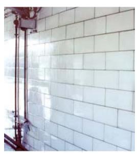
Since the early 90's, we've seen "basic" pre-faced concrete block being used quite extensively (and generally successfully) in automatic bays ... especially in oil company washes.
