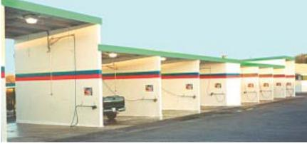
Bill Sartor transformed the walls of this tired ol' grungy 8 bay in San Antone via spray-on fiberglass. The result: bright, slick, durable, easy to clean/maintain walls that incorporate a sharp, lively blue and red "racing stripe" as an integral part of the wall coating.
