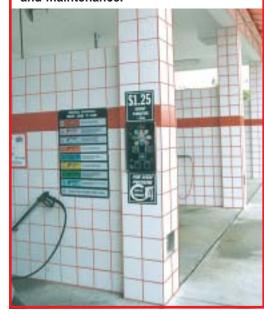
by Frey's company. He uses colored epoxy resin grout that matches the accent tile in the bay. By using the colored grout, it prevents the dirt from showing easily. The tile they use is a fired ceramic tile usually 8  $\times$  8, but recently they have been using larger 10  $\times$  10 or even 12  $\times$  12 tiles. Greg recommends using Klean Wall (see info under Spray-on Fiberglass for more detail), a mild acid cleaner to prevent etching of the tile.
