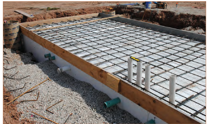
10" roof system with penetrations ready for cement.
