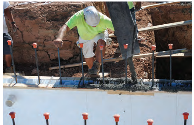
Fill FORMS with 4000# PSI cement.
