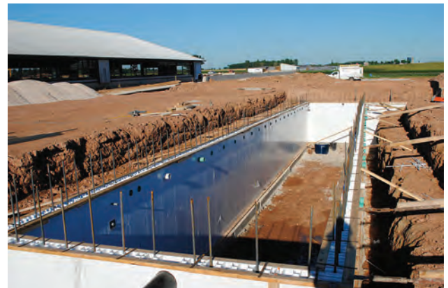
Finished shelter walls ready for floor and roof.
