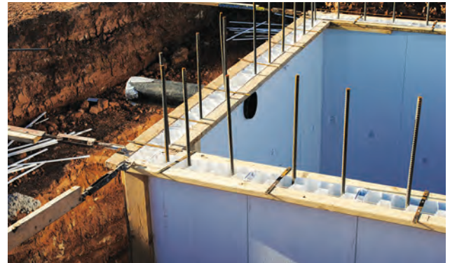
Concrete FORMS with rebar.
