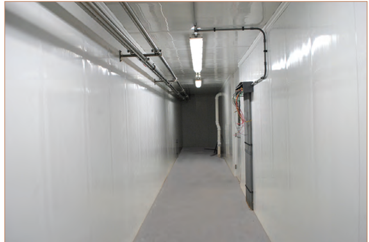
Finished Underground Shelter
