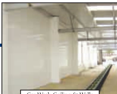
Car Wash Ceiling & Walls
