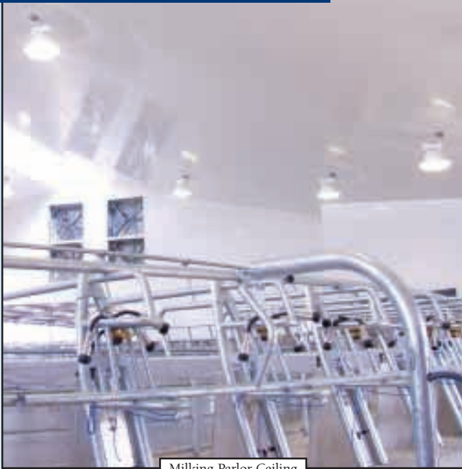
Milking Parlor Ceiling
