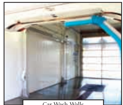
Car Wash Walls
