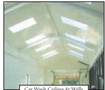
Car Wash Ceiling & Walls
