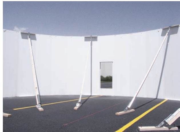
Example of Interior Bracing
