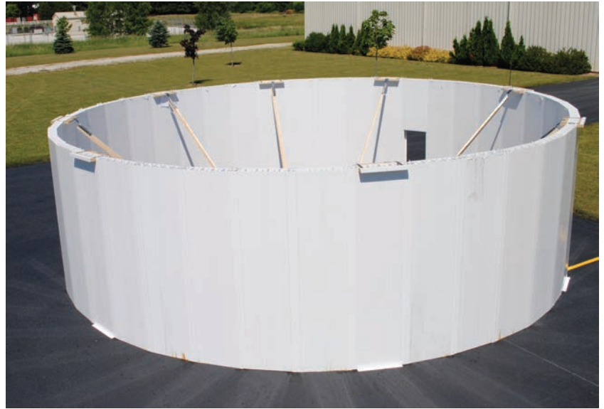
Extrutech Concrete FORM Panel Storage Tank 6" and 12" thick walls, 9' high and 30' diameter Volume = 6,361.73 gallons
