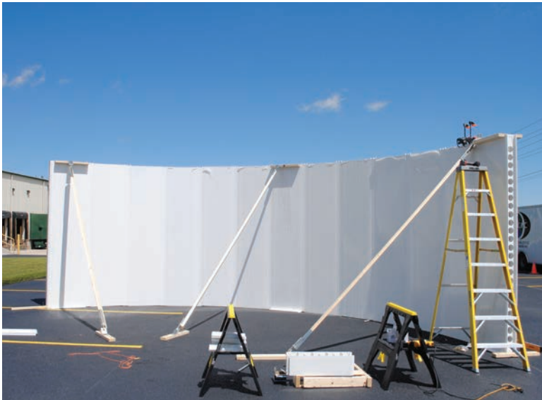
Two foot wide panels snap-together for quick installation.
