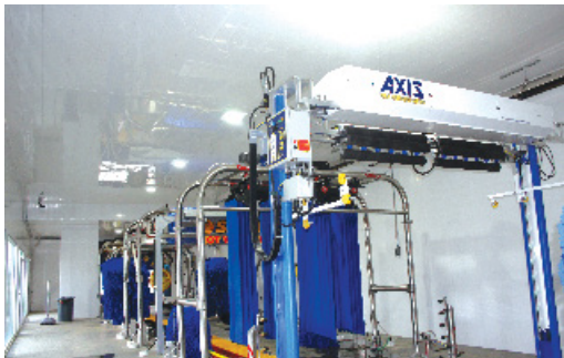
Car Wash Walls and Ceiling
