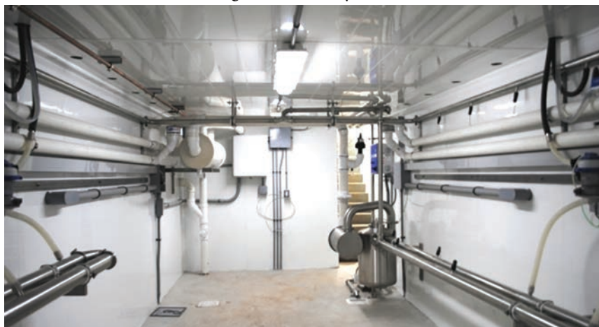
Milk Transfer Tunnel using Extrutech Stay-In-Place FORM Panels
