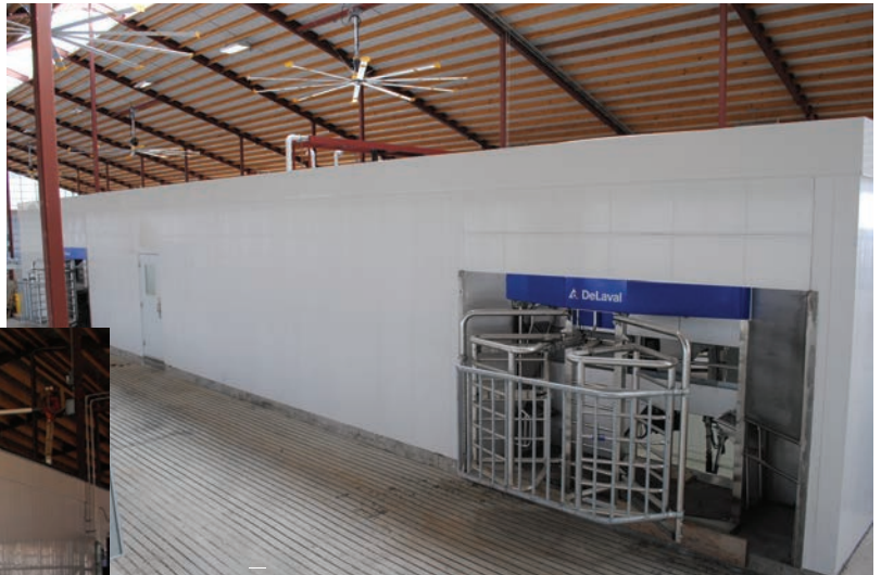
Robotic Milking Room Structure using Extrutech Stay-in-Place Concrete FORM Panels
