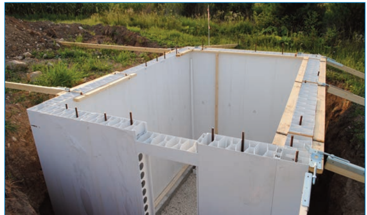
Basement walls using 8" thick Extrutech FORM system.
