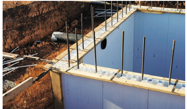
Concrete FORMS with rebar.
