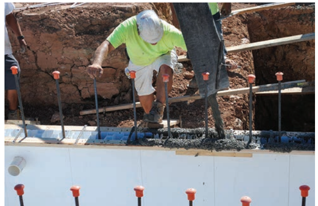
Fill FORMS with 4000# PSI cement.
