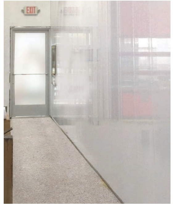
2-1/4" P224 Partition Wall Installation
