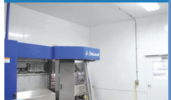
Interior of Robotic Room Walls
