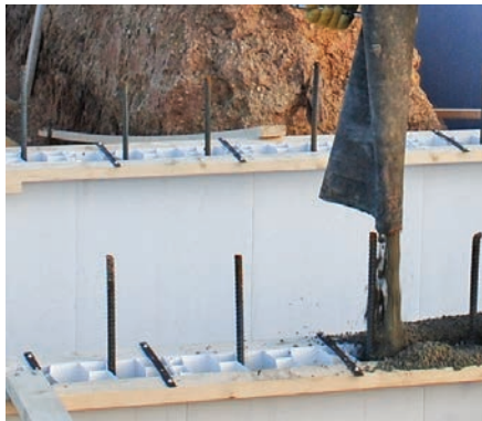
Snap together, insert splines, brace, add rebar and pour.
