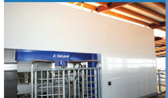
Exterior of Robotic Room Walls
